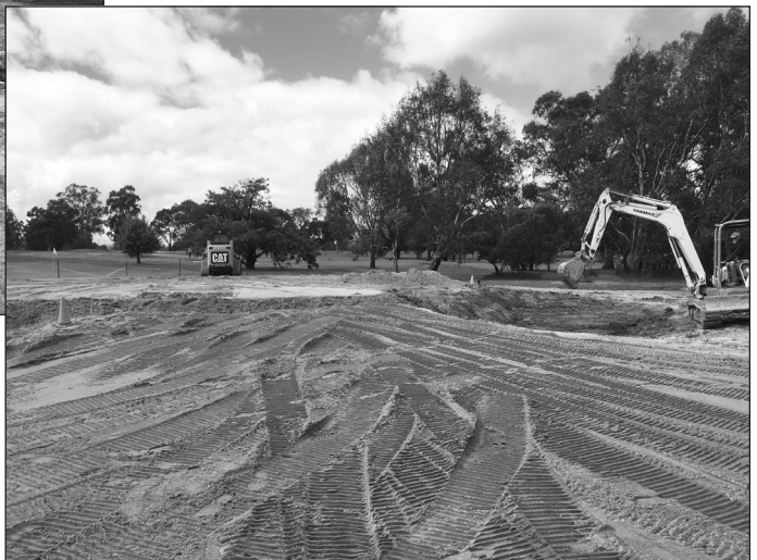
Shaping the bunkers
