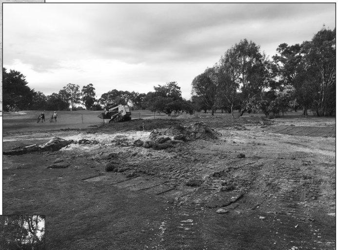
Work beginning on the new 16
