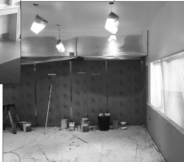
Kitchen being refurbished
