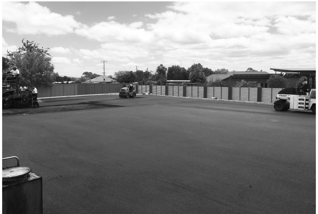
Sealing of the rear carpark
